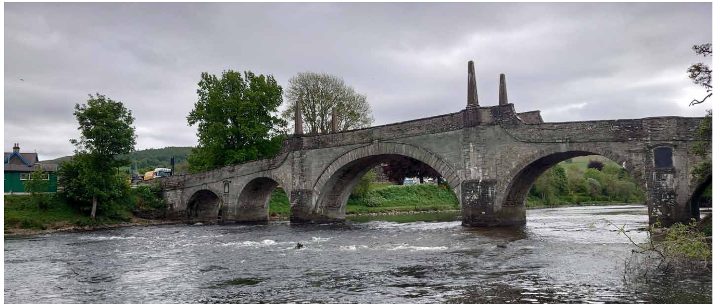
Downstream elevation from north bank.
