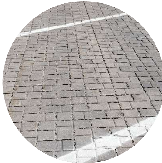
Parking - permeable paving
